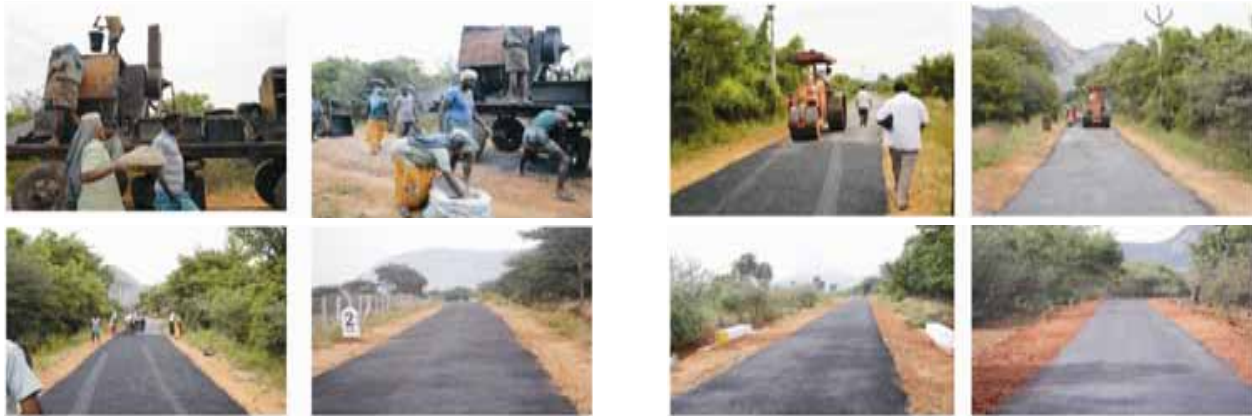
Fig 4.7: Laying of BT roads using Plastic Waste
