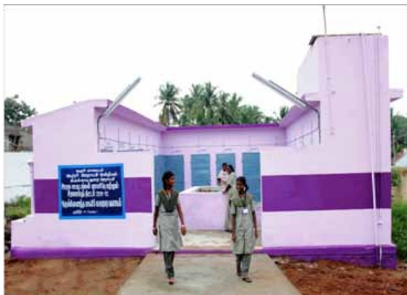
Fig. 4.6: Integrated Women Sanitary Complex
