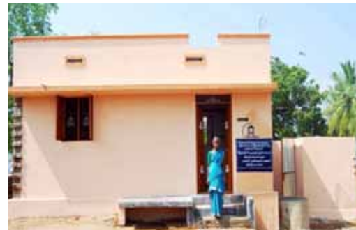
Fig.4.1: House constructed under IAY
