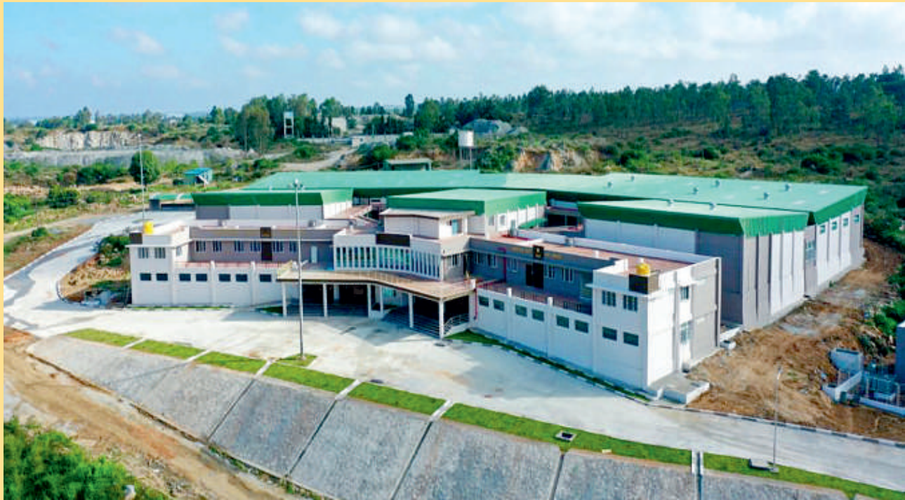
Construction of International Flower Auction Centre in Hosur with facilities to store 2.50 Lakh flower stems at refrigerated warehouse, Auction Centre, Grading Centre, Traders Centre, Cold Storage Unit of 2,000 tonnes capacity, Conference Hall and 16 Retail Outlets.
