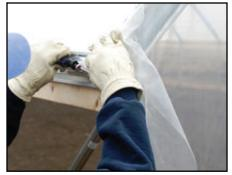
**Figure 9.** Fasten the plastic to the side or hip boards, mounted approximately 5 feet above the soil line on each side of the tunnel.
