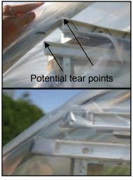
**Figure 7.** Duct tape or single-sided adhesive foam can be used to prevent plastic covering from tearing at stress points.
