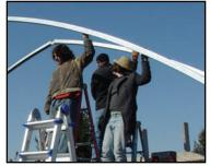
**Figure 5.** Several hands are needed to hold the metal bows or ribs while they are being installed.
