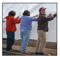
**Figure 8.** Several people located along each side make it easier to unfold and secure the plastic.
