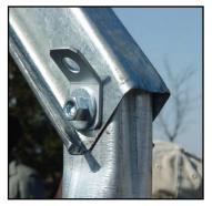
Figure 3. The metal bows are attached to the side posts.
