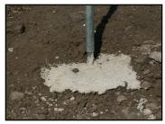
Figure 2. Post set in concrete.
