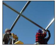
**Figure 4.** Purlins and the ridgepole connect the ribs together for support and strength.
