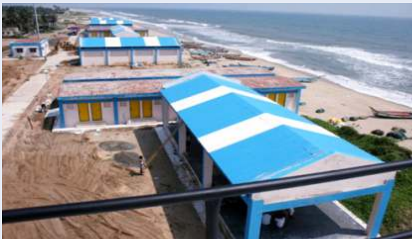
Construction of shore facilities at Cuddalore Periyakuppam Fish Landing centre under Tsunami Rehabilitation Programme(TRP).
