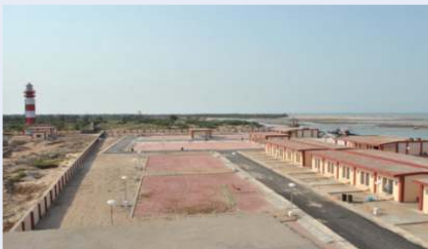
Construction of Fish Landing Centre at Parangipettai – Annankoil under Emergency Tsunami Rehabilitation Programme.
