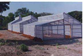
Greenhouses are framed or inflated structures covered with transparent or translucent material large enough to grow crops under partial or fully controlled environmental conditions to get optimum growth and productivity.
